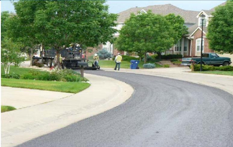
Slurry Seal is a preservation treatment applied to streets in relatively good condition to seal pavements against the harmful affects of water intrusion and environmental weathering.
