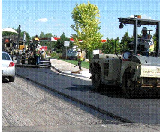
Asphalt overlay is a rehabilitation treatment consisting of mill profiling adjacent to the curb and gutter or as needed, followed by placement of a new asphalt layer.
