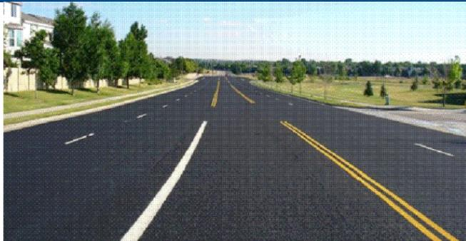
Chip Seal is a preservation treatment that is applied to streets in relatively good condition to seal pavements against the harmful effects of environmental weathering.
