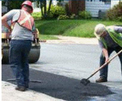
Patching of weak or failed areas extends pavement service life by preventing water infiltration into pavements which leads to accelerated deterioration.
