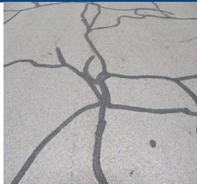
Crack sealing is a “first line of defense” pavement preservation treatment. Crack sealing prevents intrusion of water and incompressible materials into cracks to prevent accelerated deterioration of the asphalt.
